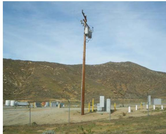
d) Closer view of SCE overhead electrical distribution and possible PV tie-in location if virtual net metering were allowed by SCE. Credit: Otto Van Geet, NREL
