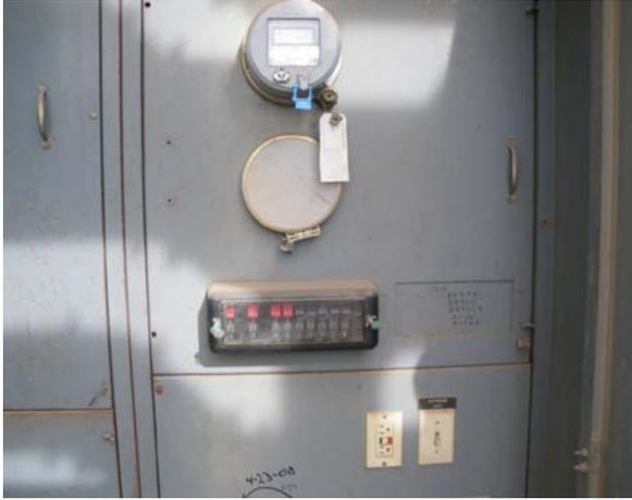
a) SCE main meter 3-029-1238-11 in main distribution & metering panel "MDP" at existing treatment plant located in center of plant.
